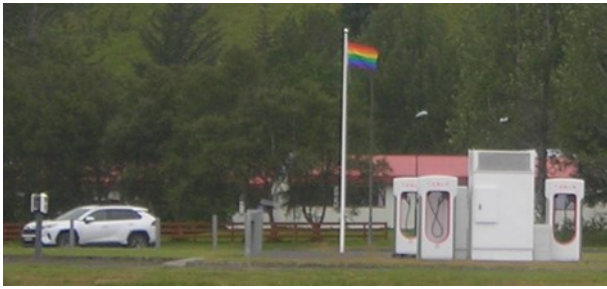
Kirkjubaejarklauster (176) - electric car charging.
